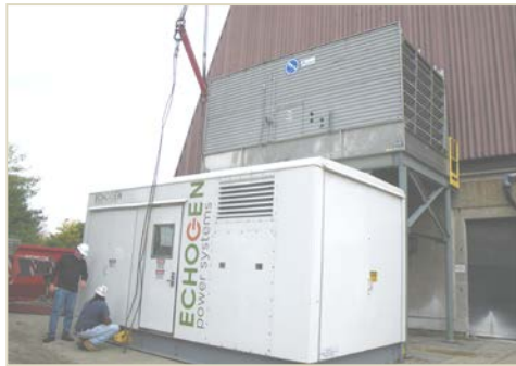
Figure 13: The 250 kWe heat engine will begin long term endurance testing at the Akron Energy Systems district heating facility (Akron, OH U.S.A) during 2Q 2012.
